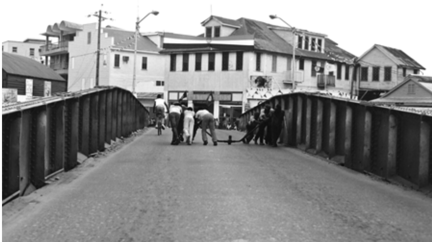
Crew starts to swing the bridge, 1986
