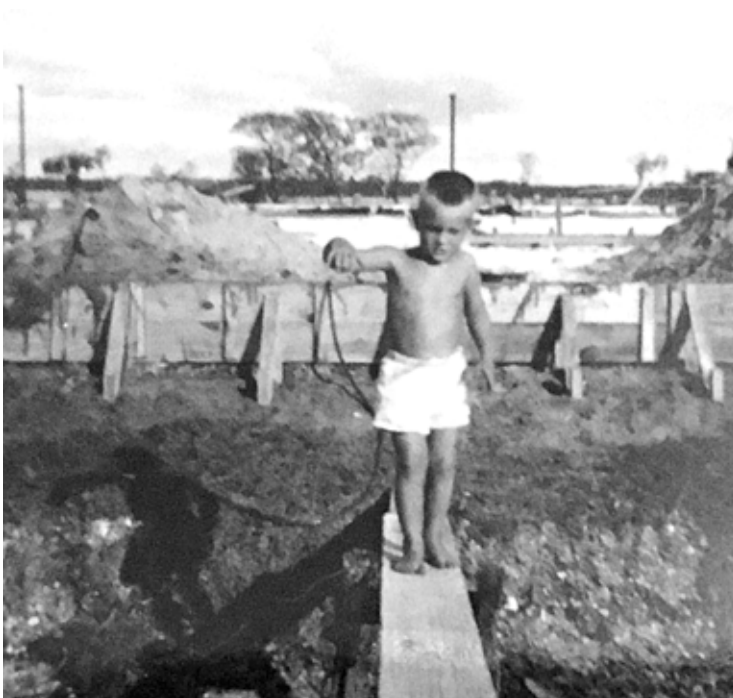
Alex on gangplank between shore and boat during construction of The Screen Cage, 1952
